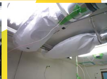
Low velocity fabric air diffuser on ceiling
