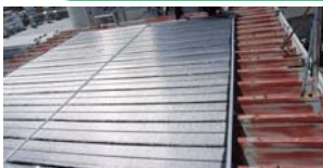
Sunshade Sheets on Folded-plate Roof
