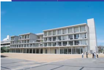
School Building with Staircase Chimney
