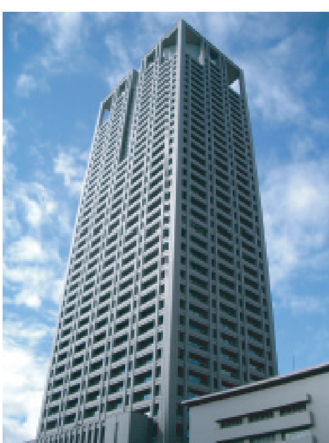
41 Stories High-Rise Office Building using This System
