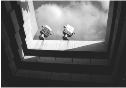
Fig. 7. Sunlight reflecting mirrors at the top of Bldg. D.
